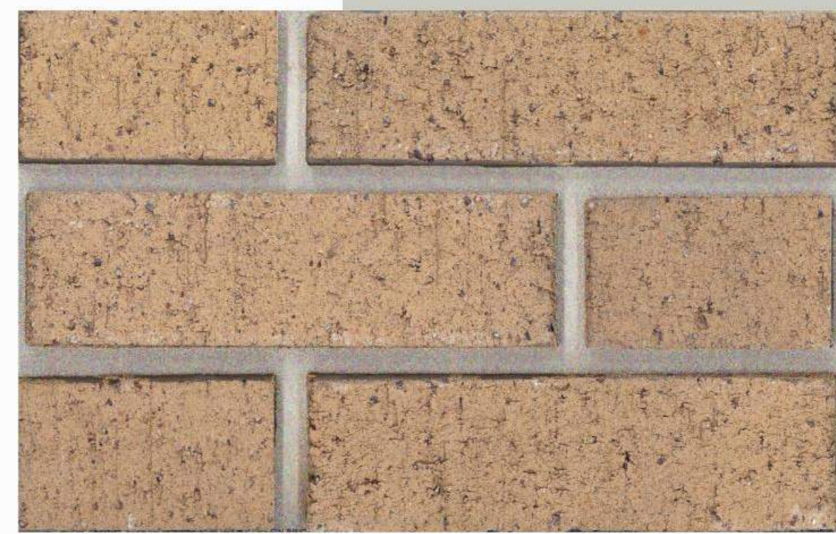
B3 - CHEROKEE BRICK "CHEROKEE ROSE" INTENDED TO COORDINATE WITH EXISTING PRECAST WALLS BEYOND
