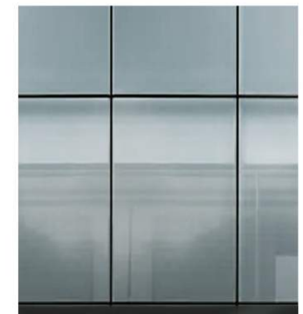
GLAZING - GUARDIAN SUNGUARD SNX CLEAR (GRAYISH) 62% LIGHT TRANSMIT / 11% REFLECT
